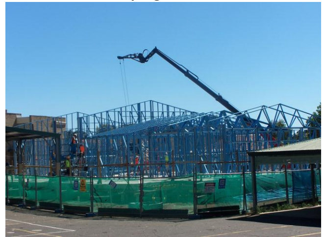
Block 5 nearing completion 4/3/2013
